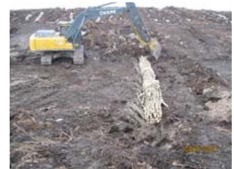
Fascine placed in west swale perpendicular to the flow of water (left). Fascine being covered with soil with excavator (right). Live stakes were placed alongside the dead fascine.
